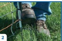
2. Install the first post or lay it on the ground with the string attached at the net's starting point. When installing the post, the step-in part of the post should face (at a 90 degree angle or perpendicular) towards the net.
